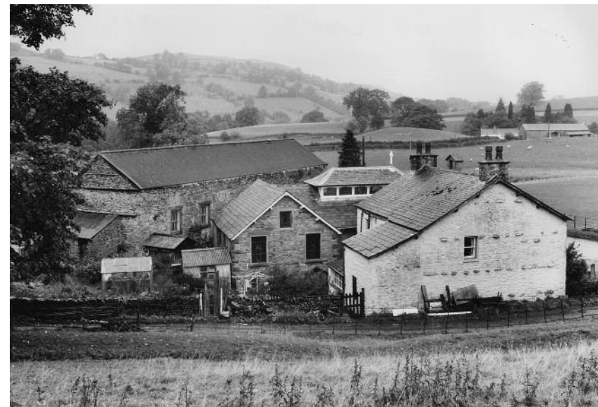
The church and surrounding buildings looking north-west towards the fells
