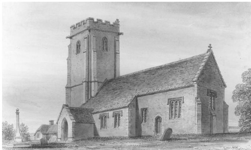
Exterior view of St Thomas's church from the south-east, by J Buckler, 1837. The view shows the chancel's late mediaeval windows before their removal. The thatched Tudor rectory is also visible. (COURTESY OF THE SOMERSET ARCHAEOLOGICAL AND NATURAL HISTORY SOCIETY)
