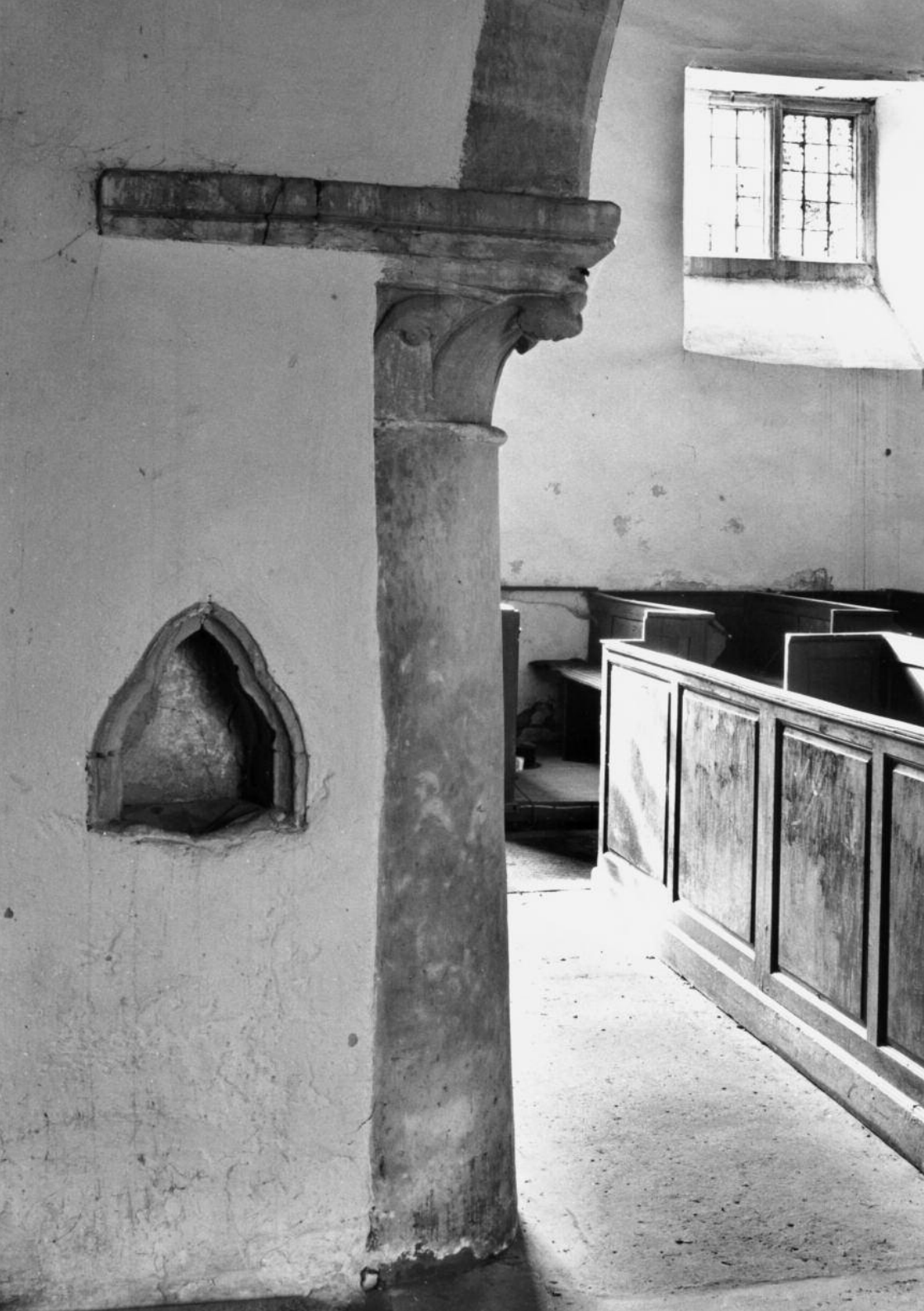
North aisle piscina, 12th-century arcade and 'domestic' window in the south wall (Christopher Dalton)
