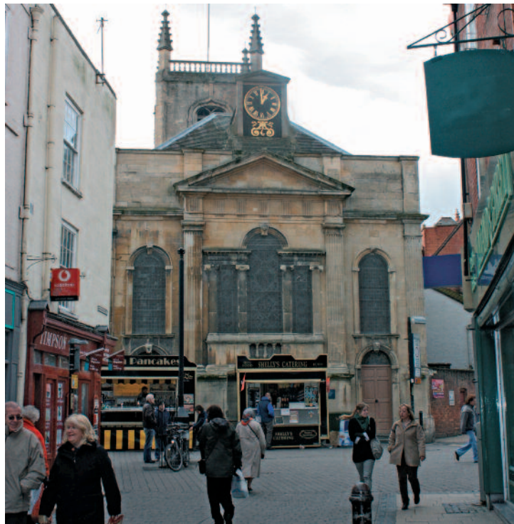
Left: East end of church from Mealcheapen Street Right: West tower
