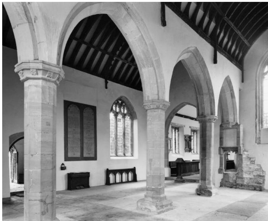
Interior looking north-east showing the arcade
